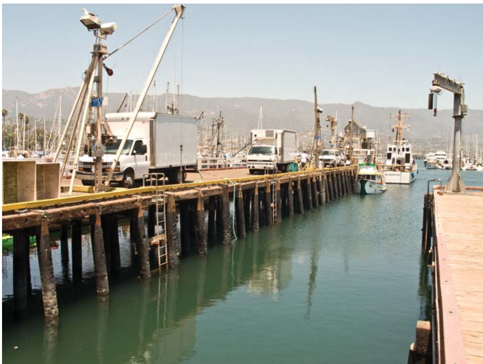
OSHA standards require some method of hoisting an unconscious or injured diver out of the water, no matter where you are working. Trying to haul an unconscious diver even a short distance from the water may be impossible without the right equipment or enough manpower.
